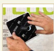
Weathertight sealing grommets for cables and pipes that penetrate the weathertightness layer.
